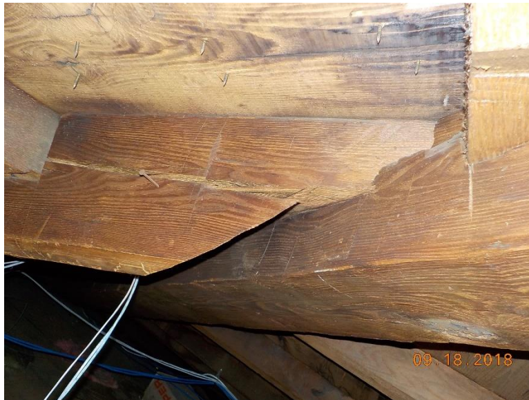
Figure No. 10 – Close Up View of Typical Horizontal Shear Failure at the Bottom of Tenon Cut Top Ends of an Infill Roof Beam at the Flush Framed Connection at the Side of the Main Roof Hip Beam
