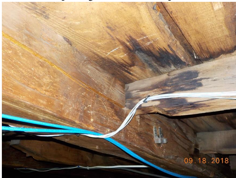
Figure No. 14 – Typical Horizontal Shear Failure of a Main Roof Beam at the Bottom of Mortise Cuts for Flush Framed Connections With the Tenoned End of a Typical Roof Purlin
