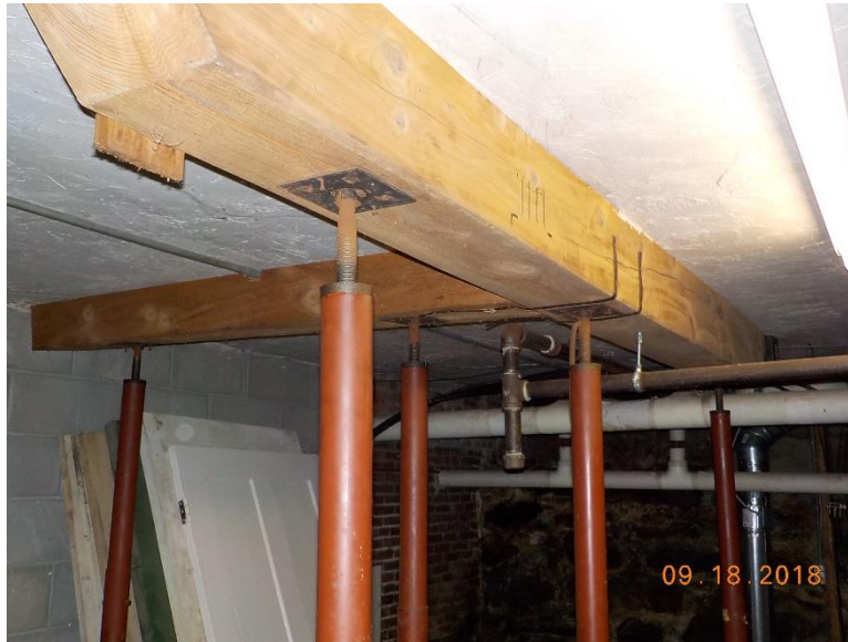
Figure No. 3 – Basement Level Temporary Timber Reinforcement Floor Beams and Temporary Adjustable Steel Shoring Posts
