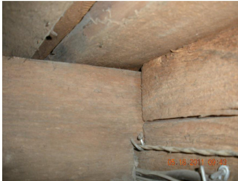
Figure No. 7 – Anticipated Timber Framing Connection Damage at the Side of the Main Stairway Floor Opening at the 2 nd Floor Level
