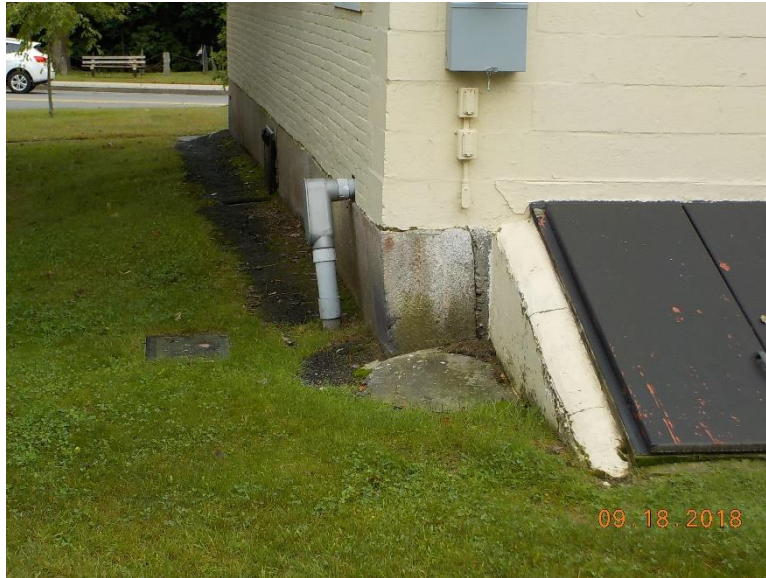
Figure No. 1 – Rotated Cut Stone Piece in the Sidewall Foundation
