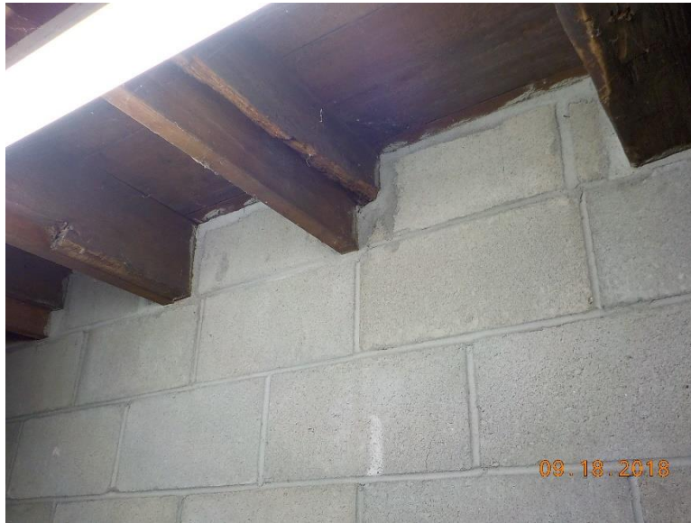
Figure No. 5 – Timber First Floor Framing in Direct Contact With CMU Masonry Wall Construction at the Basement Level
