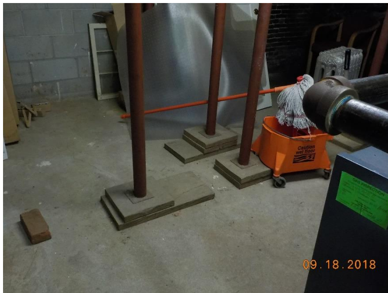
Figure No. 2 – Base of Steel Basement Pipe Columns Supported on Wood Blocking on Top of the Basement Level Concrete Floor Slab
