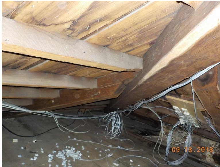
Figure No. 9 – Typical Horizontal Shear Failure in Infill Roof Beams at the Bottom of the Mortise Cuts at the Flush Framed Connections with Roof Purlins at Each Side of the Main Roof Hip Beams
