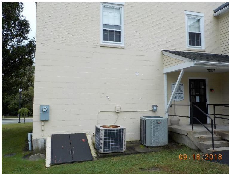
Figure No. 4 – Exterior First Floor Level CMU Masonry Bearing Wall at the Rear Wall of the Starbard Building
