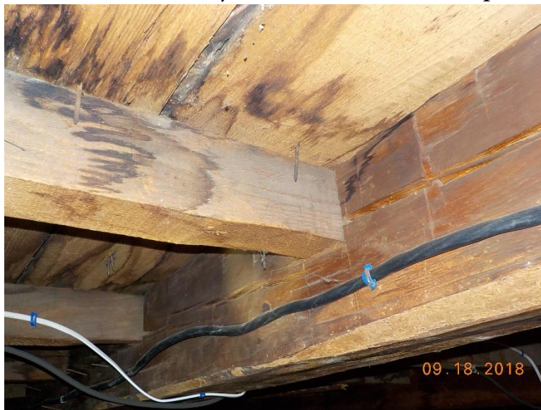
Figure No. 11 – Close Up View of Typical Horizontal Shear Failure at Bottom of Mortise Cuts at the Side of an Infill Roof Beam at the Flush Framed Connection with a Roof Purlin Adjacent to a Main Roof Hip Beam
