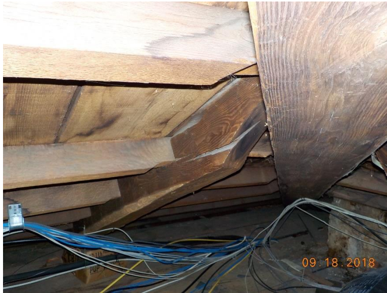
Figure No. 11 – Close Up View of Typical Horizontal Shear Failure at Bottom of Mortise Cuts at the Side of an Infill Roof Beam at the Flush Framed Connection with a Roof Purlin Adjacent to a Main Roof Hip Beam
