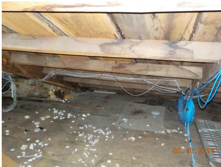
Figure No. 8 – Typical Timber Roof Framing Configuration of Main Roof Beams and Horizontal Roof Purlins Spanning Between the Roof Beams
