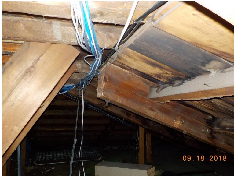
Figure No. 13 – Typical Horizontal Shear Failure of Main Beam at the Bottom of Mortise Cuts for Flush Framed Connections With Roof Purlins at Side of Roof Opening for the Roof Cupola
