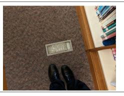
271 Floor Box Cover Issues (Pod Commons) *Pod commons* - Existing floor boxes have plastic covers that break. Staff has been removing them in pods when reflooring.
