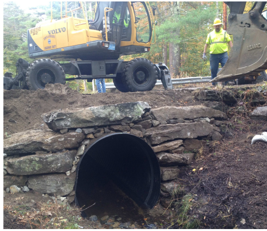
Reservoir Street culvert upgrades
