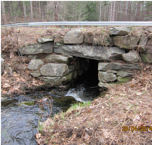
Reservoir Street stone box culvert
